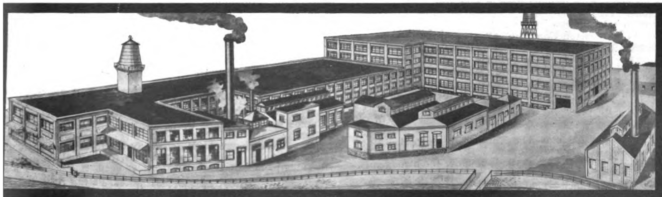
View of the complete new plant of the New Process Raw Hide Company, Syracuse, N. Y., including the recent additions
